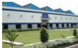
Flow Equipment factory, Sarole
